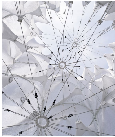
Fig 1: Interior photo of Hybrid Tower. A 9m tall form-active hybrid structure (CITA/KET 2015)
